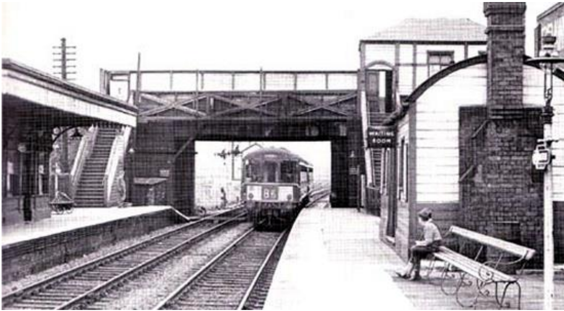
The original Darlaston (James Bridge) Station which closed in 1965
