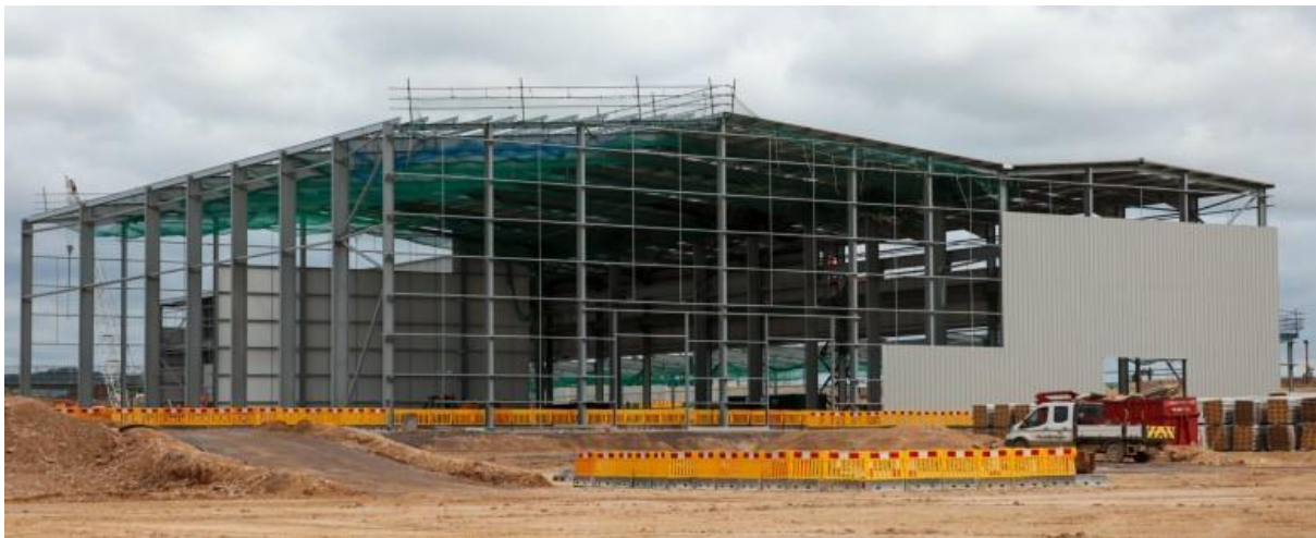
The new precast tunnel segment factory.
