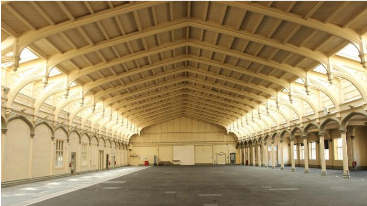
The passenger shed of Brunel's Old Station in Bristol.
