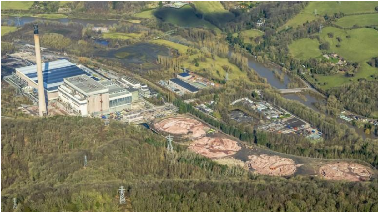
The undeveloped site after the demolition of the four cooling towers (Shropshire Star)
