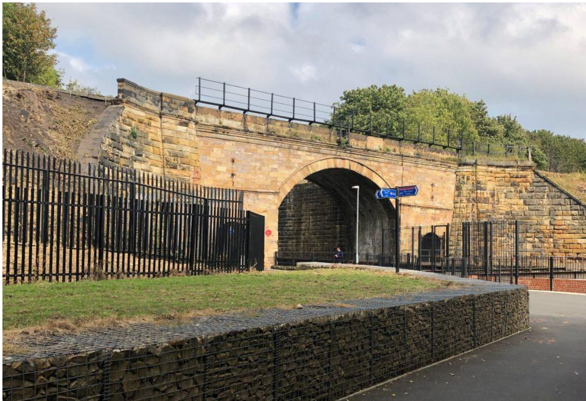
The Skerne Bridge
