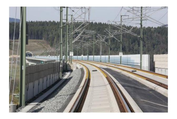
HS2 Ltd said the use of modular slabs would reduce maintenance costs and improve performance compared to ballasted track. More than 780 km of Porr's slab track has been installed worldwide, with the first section at Langenlebern in Austria having been in use since 1989. It has been widely deployed in Germany, including on the north-south and east-west routes at Berlin Hauptbahnhof, and on the Berlin – Erfurt – Nürnberg high speed line.
