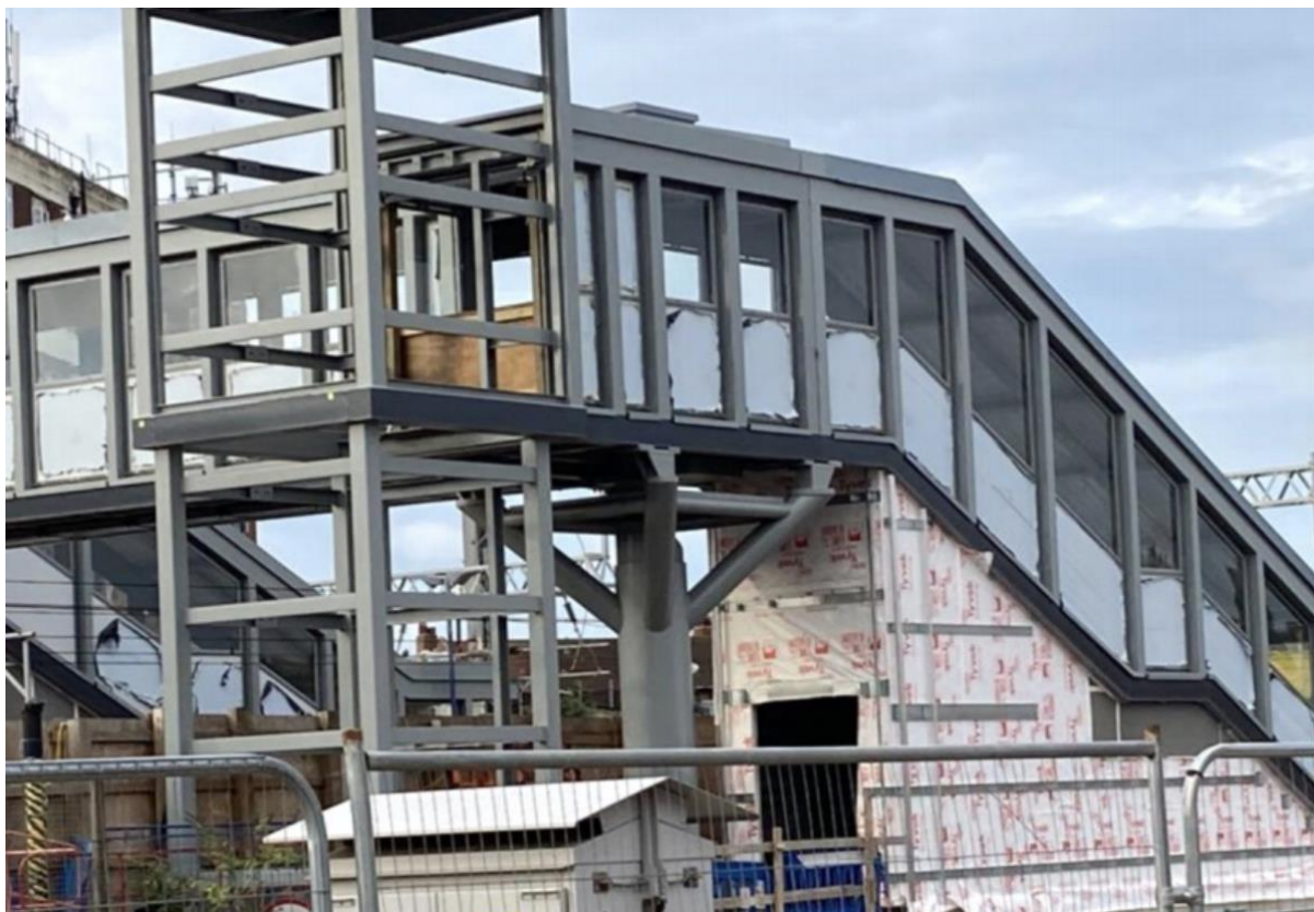
Walkways have been completed at Acton Mainline Station
