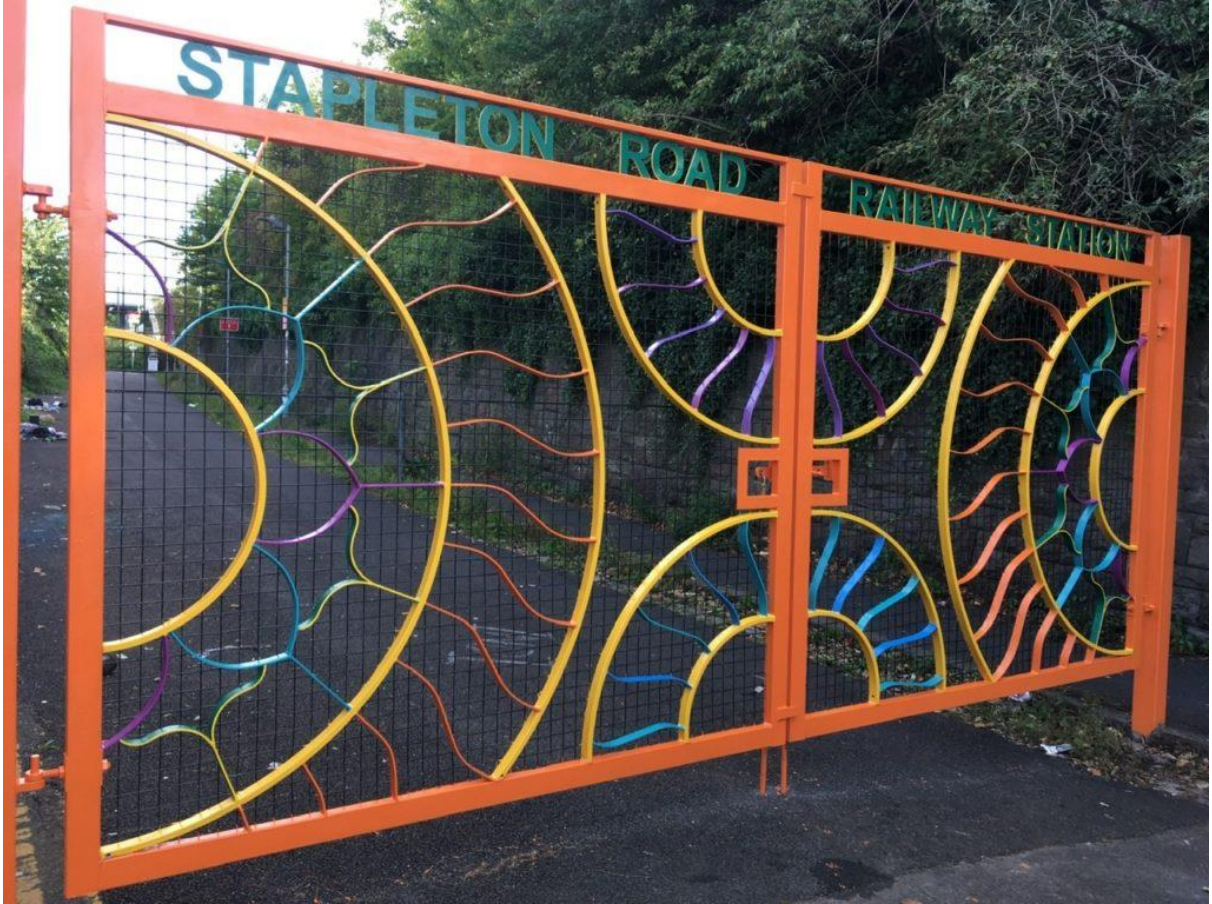
The new gates have brightened up the entrance to the station (Mary Reynolds)
