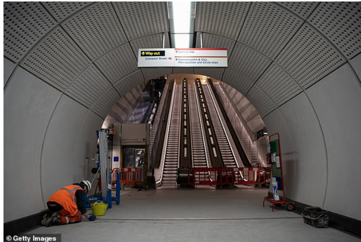
(An access corridor within Liverpool Street Crossrail station in February 2020)
